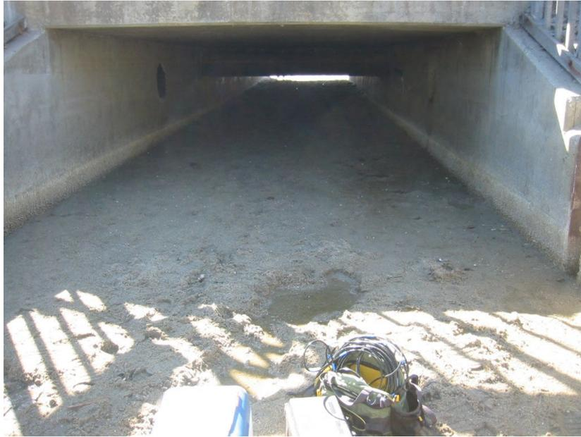
**Figure 3.9. Moran Lake Box Culvert Closed with Sand– October 28, 2003**
