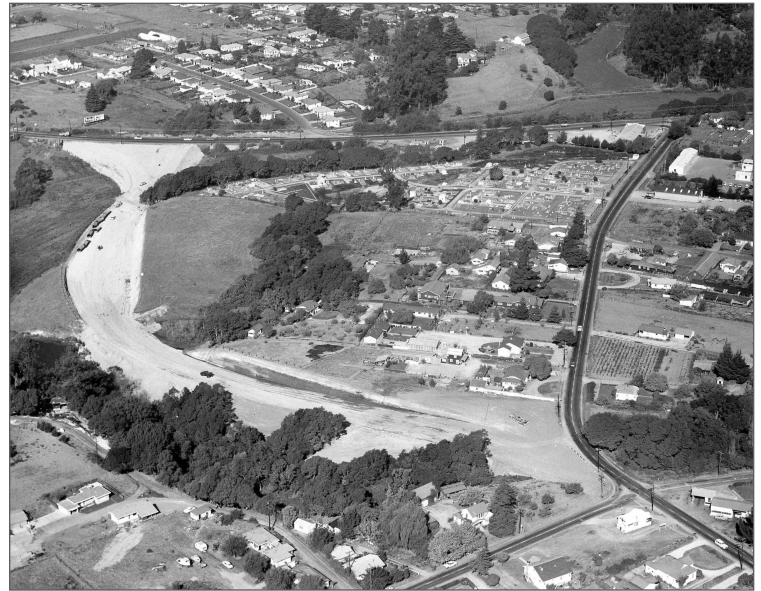
1959 Cut-and-fill Capitola Road project connecting Soquel Avenue at “Slaughterhouse Curve” (upper left) with 7 th Avenue (lower right). The original Lower Soquel/Capitola Road is on the right—now Capitola Road Extension. (Courtesy of Covello and Covello Photography)
