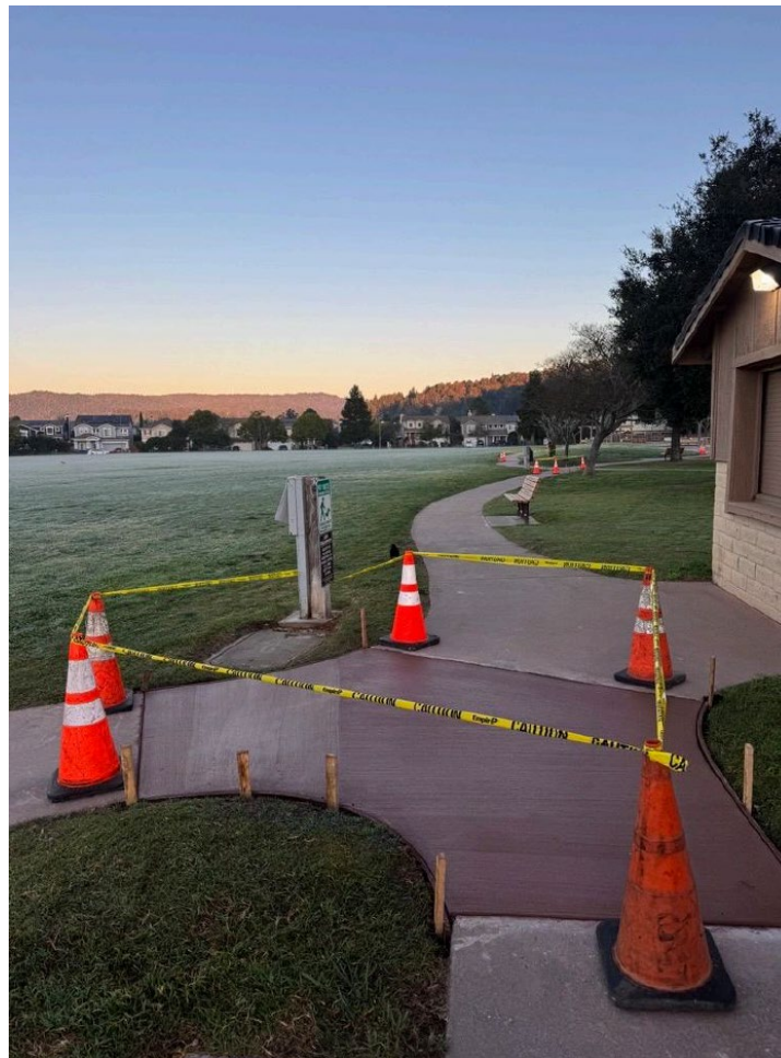
Skypark repairs, City of Scotts Valley
